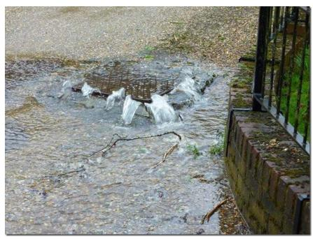
rainfall the sewer is overloaded and the manholes lift. Anglian Water confirmed that this <u>cannot</u> be solved as a larger sewer would result in the flows being too slow under normal conditions, resulting in odour and blockages. 24 new houses will discharge into the system thereby increasing the amount of sewage and reducing the capacity for the surface water rain. The sewage in the system will be more concentrated and therefore more polluting.
