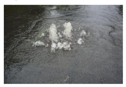
In Low Road, at times of heavy rainfall the sewerage manhole covers lift and raw sewage goes over the road and into gardens and also runs back into the stream (the Beck) to be dissipated further.
